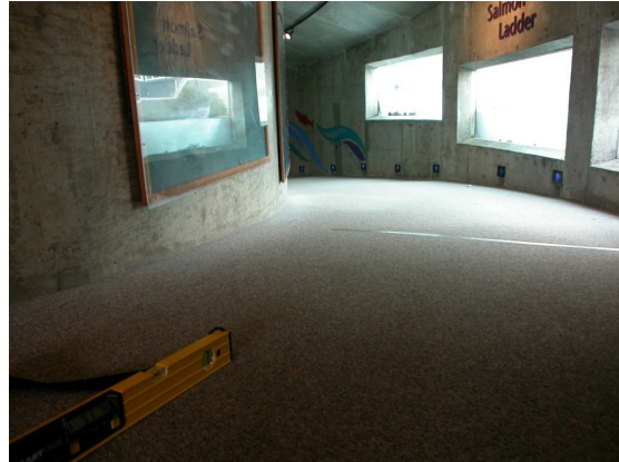
Figure 4: Steep Curved Ramp near Salmon Ladder
